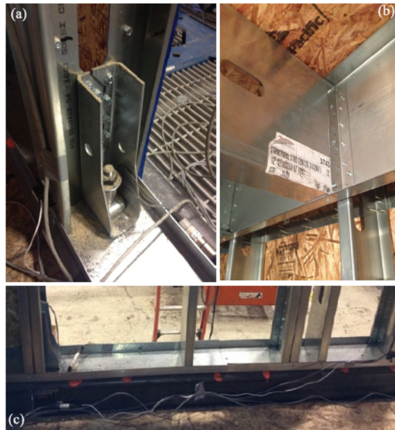
Figure 5-1. Cold-formed steel wall details
